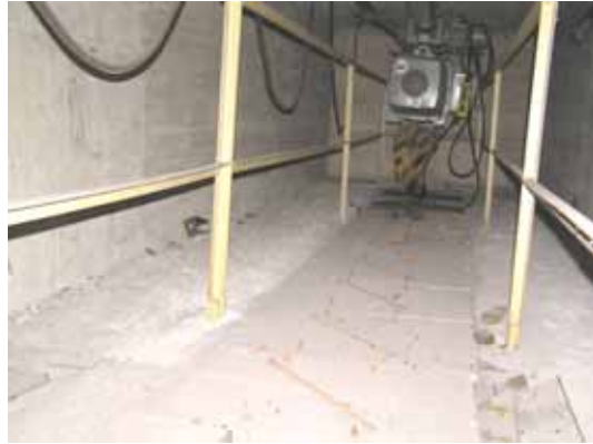
Figure 2: The hoist positioned over the chamber roof
