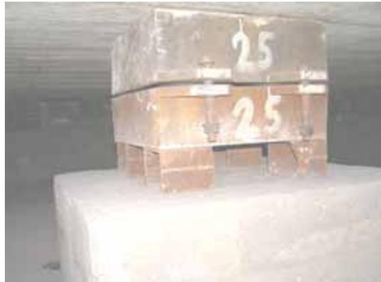
**Figure 3:** The housing with springs located in the central point of support
