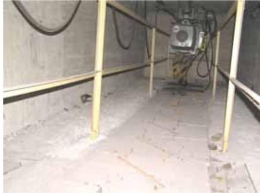
**Figure 2:** The hoist positioned over the chamber roof
